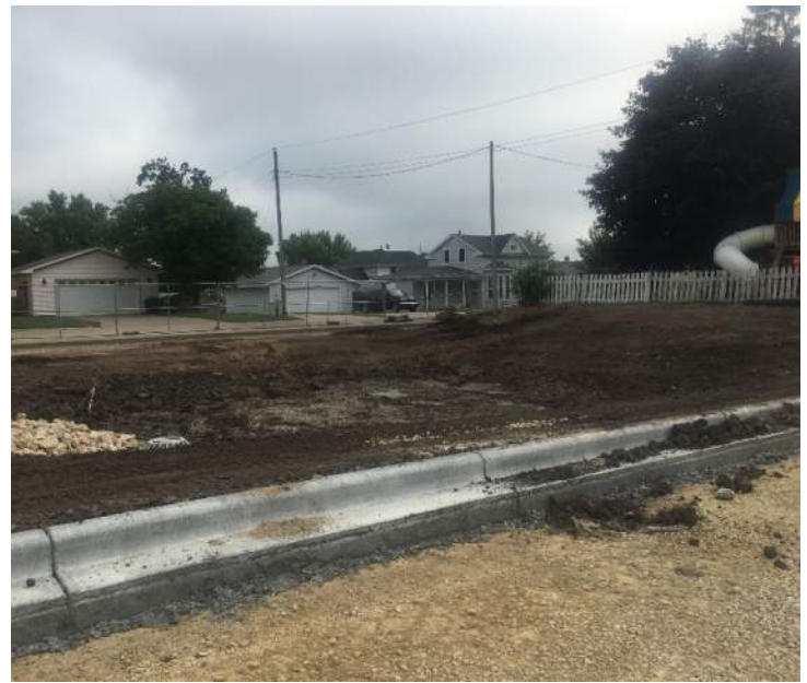
The new retention ponds that will be located to the north of the parking lot. These will take final shape in the next few weeks.
