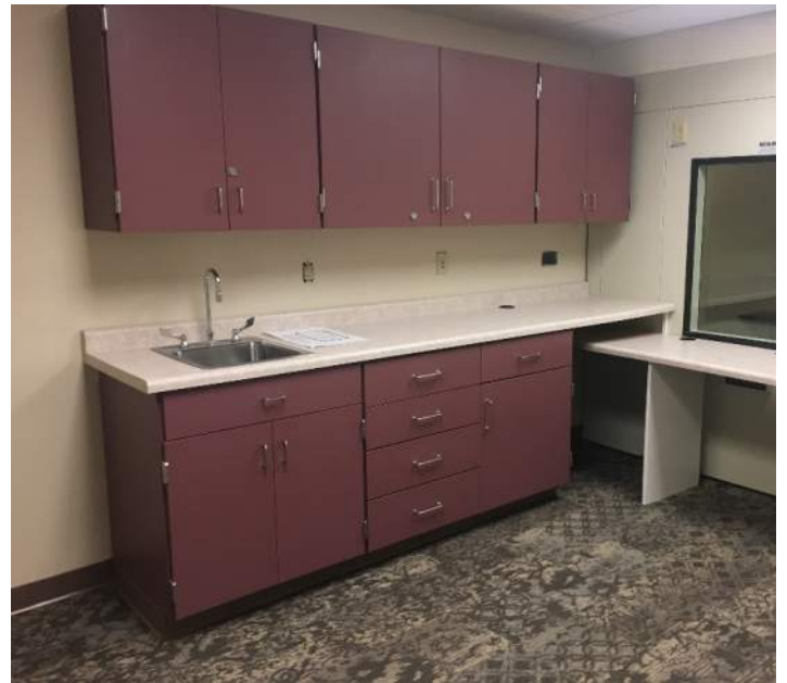
After the booth is installed, paint, flooring, and countertops and cabinets are installed. Almost ready to open for business!
