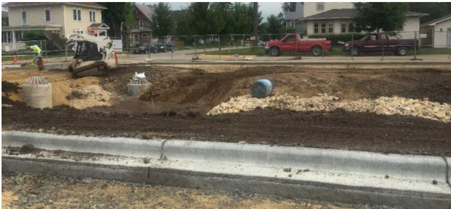
The new retention ponds and curb and gutter for the new parking lot are coming together nicely.
