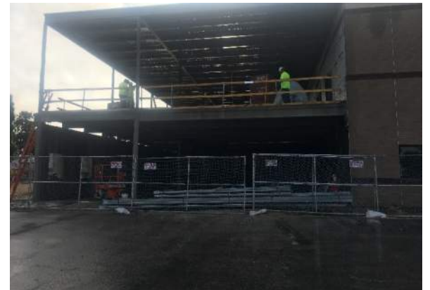
The new electrical room has the wall framing up, and will soon be drywalled and painted.
