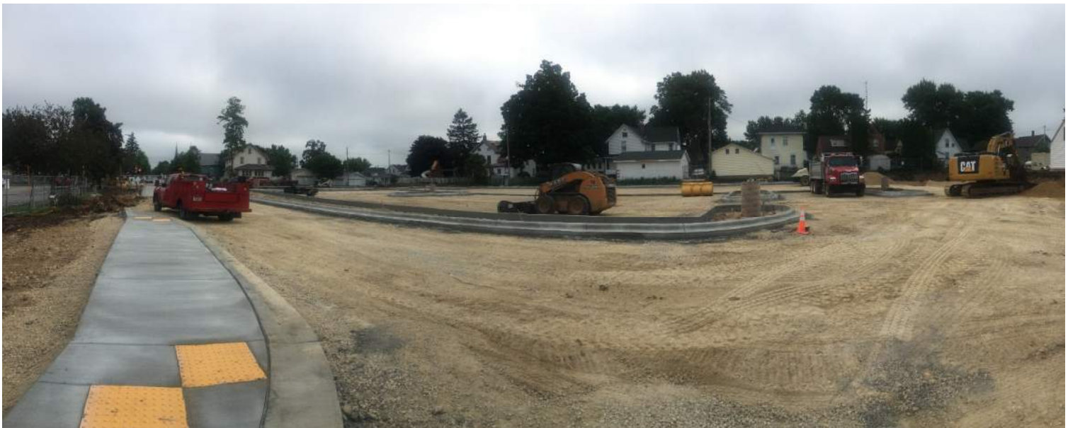
A panoramic view of the parking lot being worked on before it can be asphalted, striped, and opened up for use! The curb and gutter as well as part of the sidewalk can be seen above.
