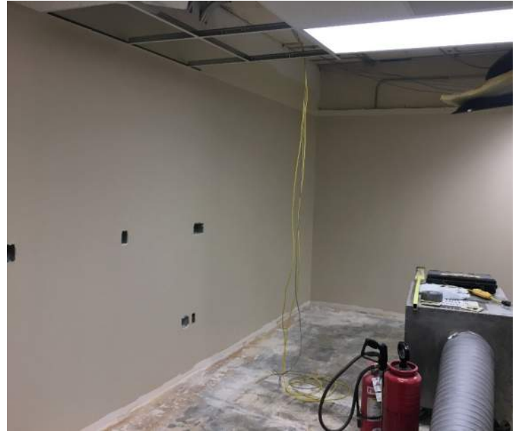
The walls and ceiling are prepped for the install of the booth. The ceiling grid and tiles are removed to allow for the booth to be installed and connected as needed.
