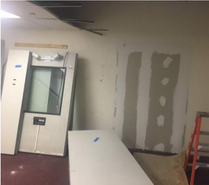
First stage of the Audiology Booth move – demolition! The area on the wall with unfinished drywall is where the booth used to sit.
