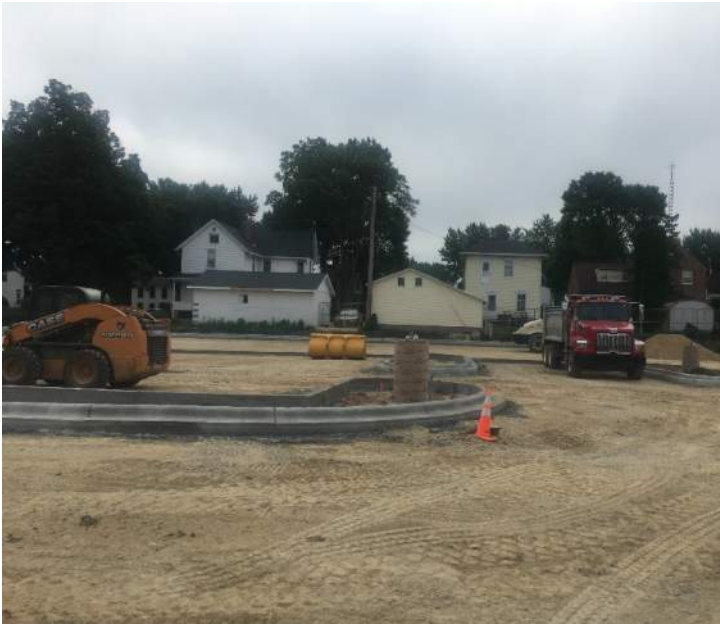
Curb and gutter being installed in the new parking lot. The asphalt and then the striping are the next steps in the process.
