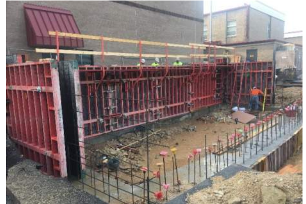
The new generator enclosure walls and footings being poured into place.
